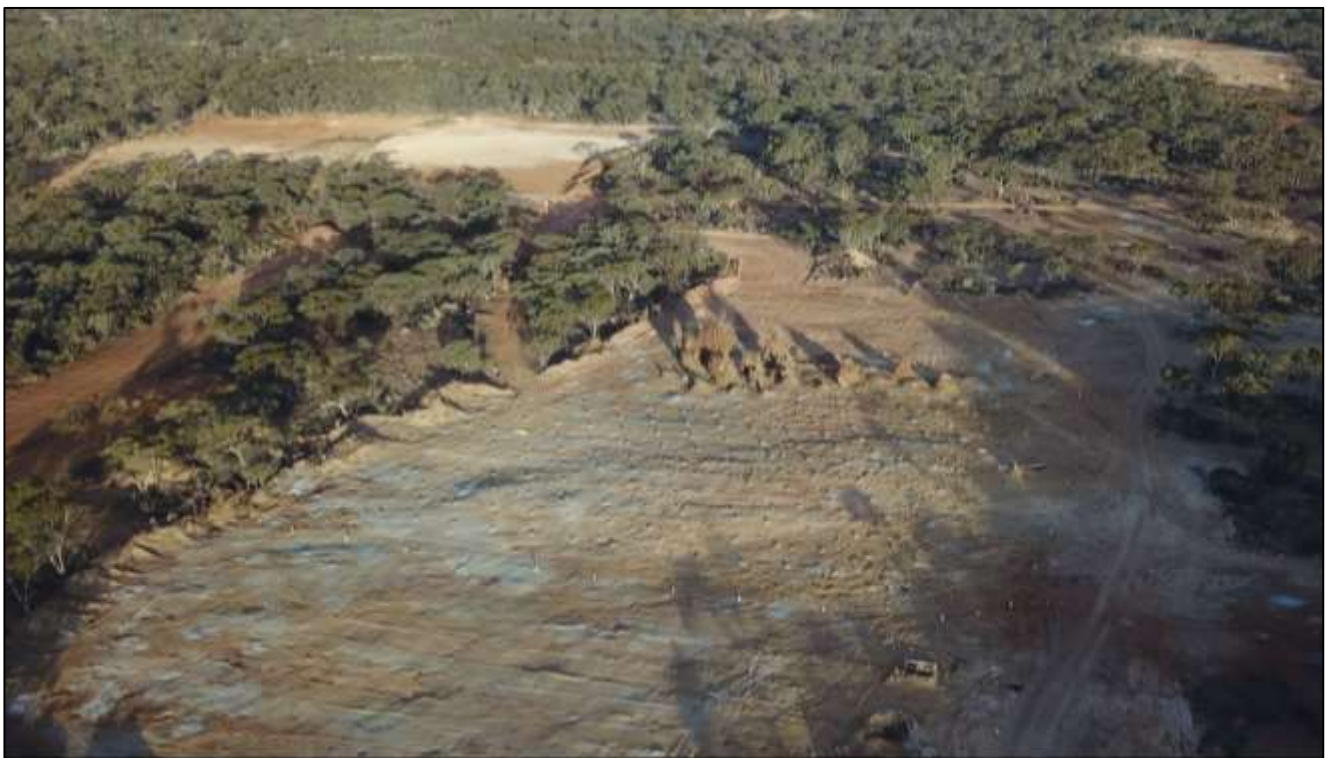
Photo 1: First blast for Widgiemooltha Gold Project at the Flinders Main pit (photo taken by Red Sparrow Drone Services)
