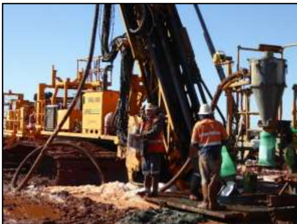
Photo 1: Lake Roe Lake RC Drilling
