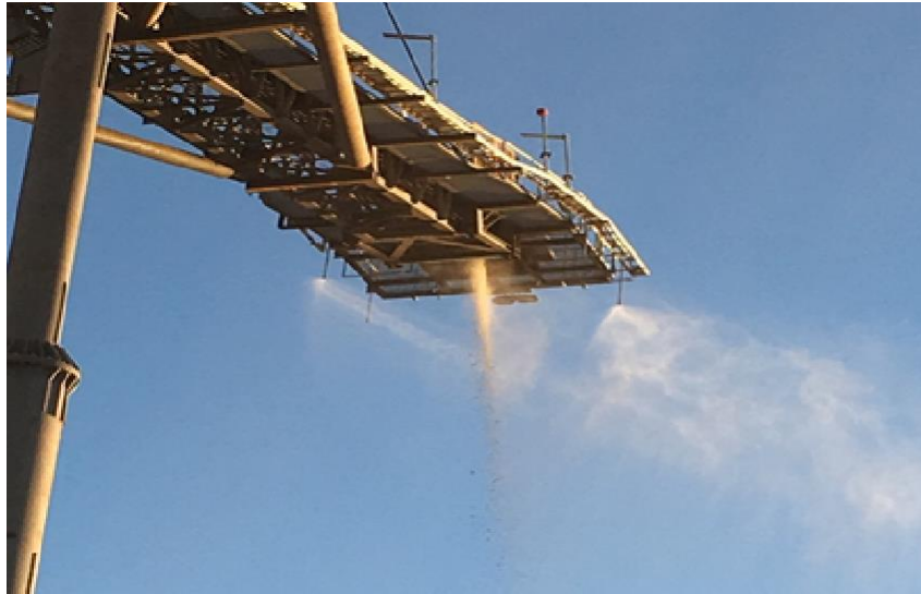
Ore Load Commissioning at Crushing Facilities - Conveyor Product Discharge (Figure 2)
