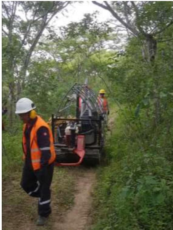
*Photo 1: Transporting components of the drill rig to site using motorised trolleys along existing tracks*
